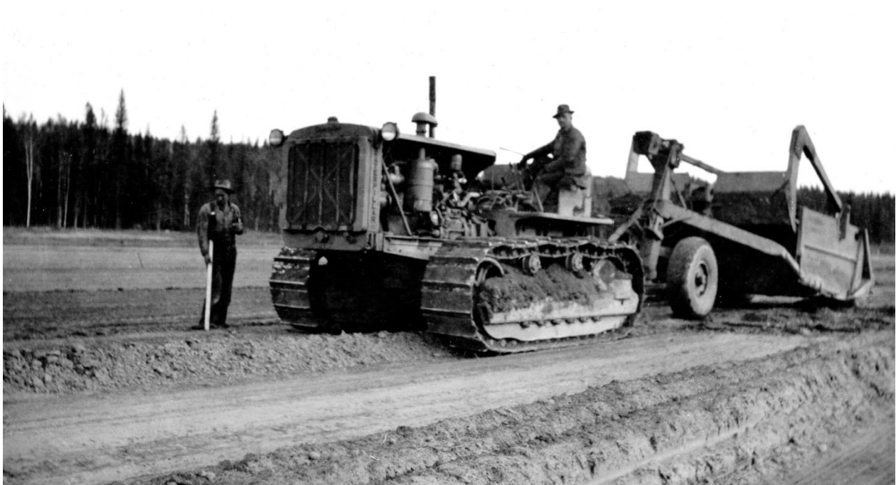
Construction of airport runway, 1959. Photo courtesy of Quesnel Museum & Archives
